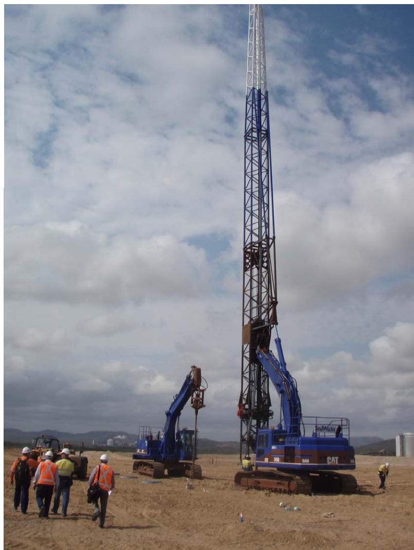
Commencement of Wick Drain installation to LNG Train 1.
