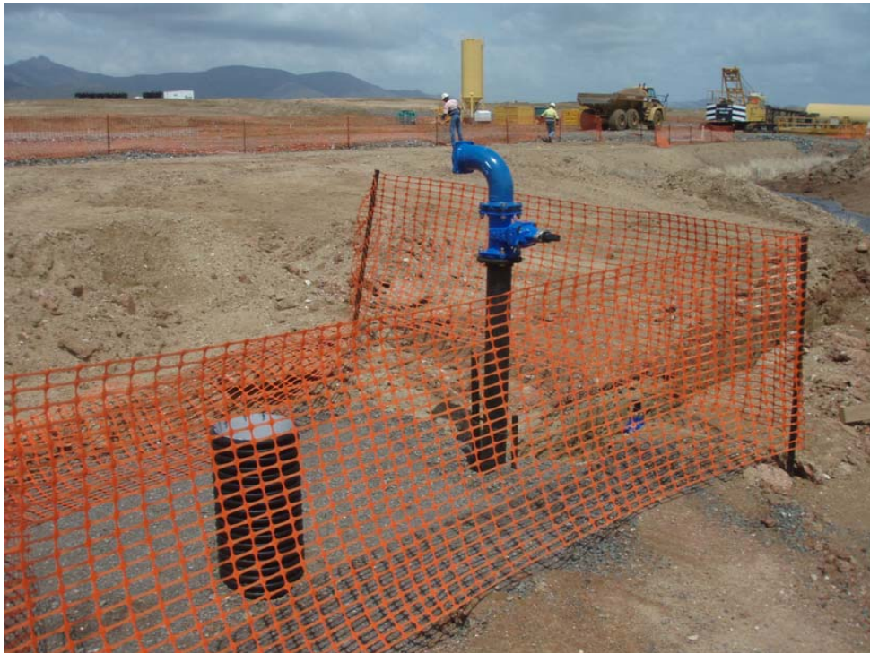
Connection of Raw Water supply to site for CSM works.
