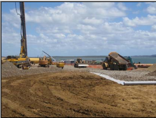
Figure 1: Formation of platform for erection of the permanent batch plant
