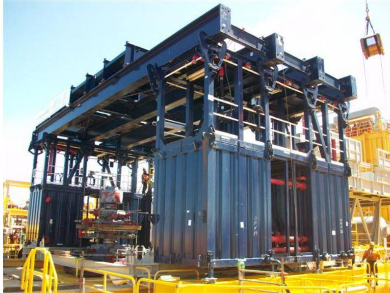
Workover unit being constructed on wellhead platform
